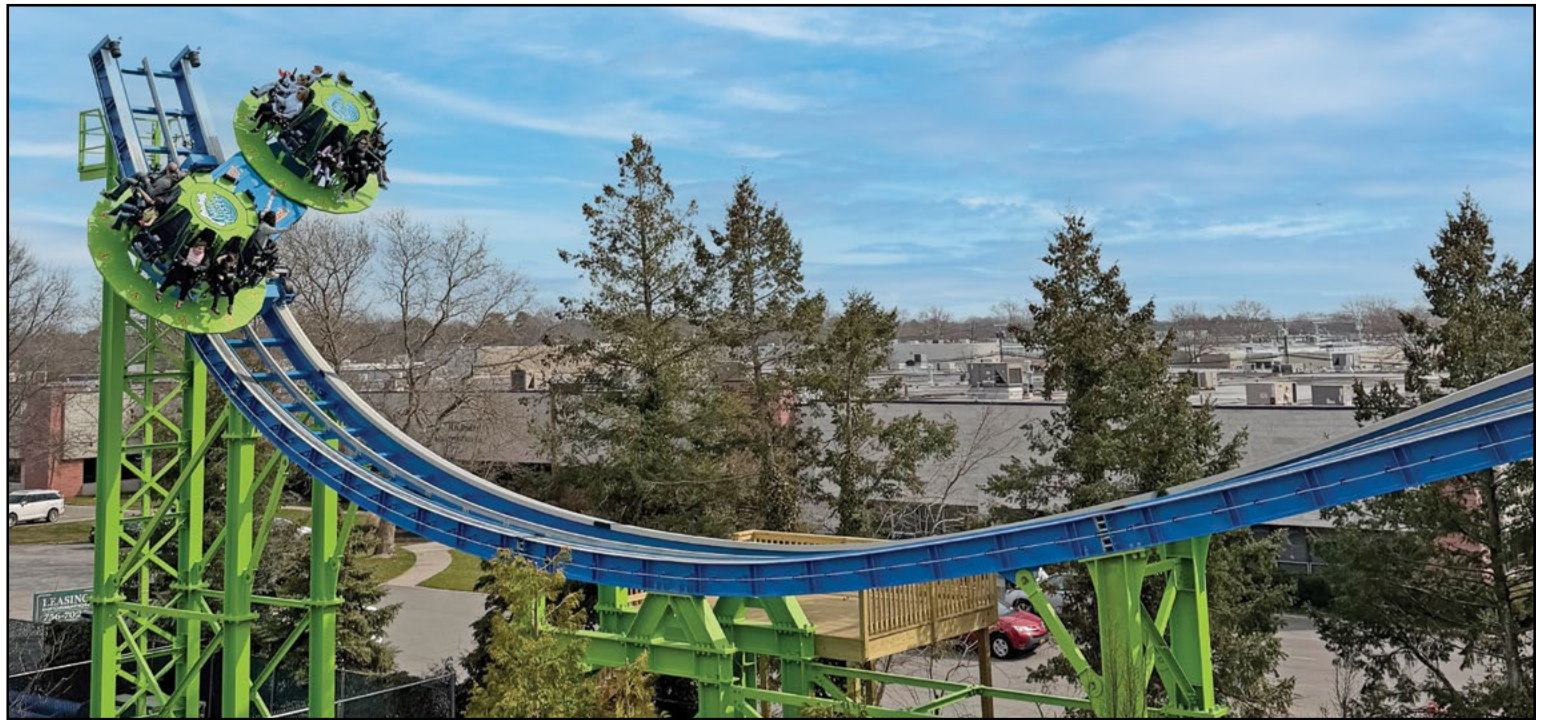
Cantilevered over the track, the rotating beam offers riders continuously changing views. COURTESY ADVENTURELAND
