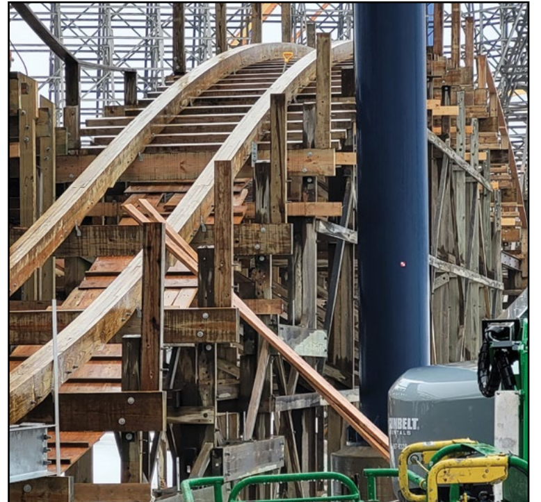
The Gravity Group's Engineered Pre-cut Track adds strength and durability to the course. COURTESY THE GRAVITY GROUP
