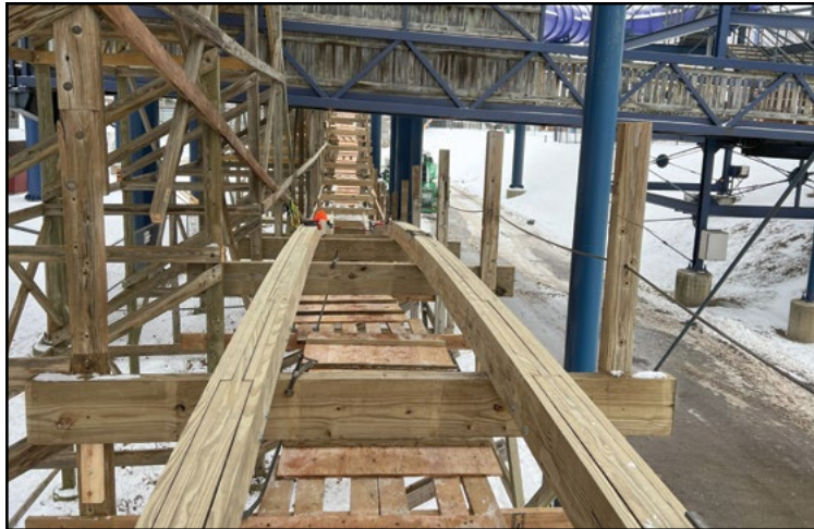
The Gravity Group's Engineered Pre-cut Track adds strength and durability to the course. COURTESY THE GRAVITY GROUP
