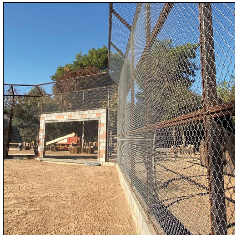
The Wildlife World Zoo's new tiger exhibit is expected to open this spring and features two mirror image habitats with common sleeping rooms behind a waterfall (above). A stainless steel woven cable, oxidized black has been used for the netting. The panels, from A-to-Z Netting in Tucson, Arizona, were chosen for their exceptional strength and durability and to enhance visibility. AT/GARY SLADE
