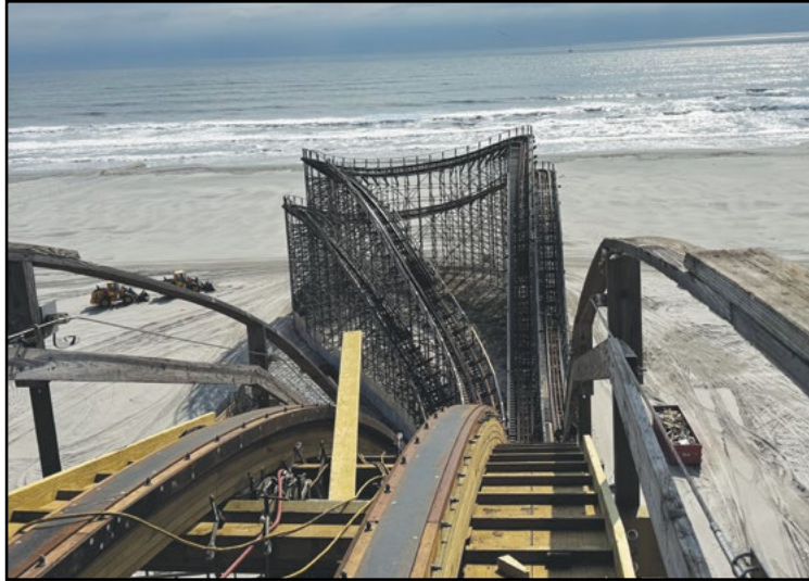
Great Coasters International Inc. not only supplied two new trains (right) for the Great White at Morey's Piers, it also re-tracked the lift hill (above) adding a layer of Ipe on the top layer. COURTESY GCII
