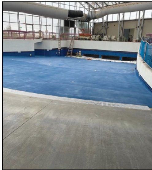
The Coat Your Pool thermoplastic surface is seen being installed on the Water-Zoo wave pool (above left). Water-Zoo also coated its lazy river. COURTESY COAT YOUR POOL
