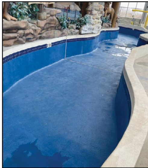
The Coat Your Pool thermoplastic surface is seen being installed on the Water-Zoo wave pool (above left). Water-Zoo also coated its lazy river. COURTESY COAT YOUR POOL
