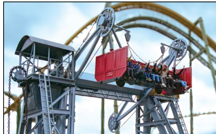
The park designed a 19th century loading crane to thematically fit into the area. COURTESY ART ENGINEERING
