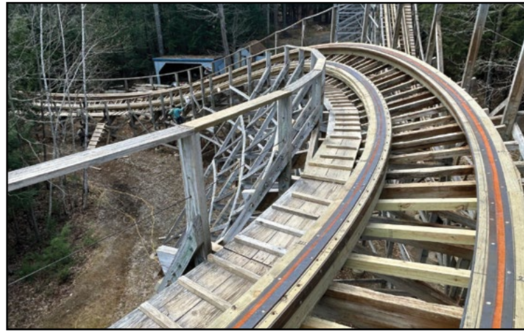
Funtown management report the off-season track work has increased the speed of Excalibur. Major curves received needed attention (above middle). In addition, Excalibur's first drop (above right, below) received precut track from The Gravity Group. COURTESY FUNTOWN SPLASHTOWN U.S.A., THE GRAVITY GROUP
