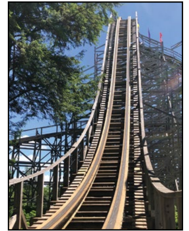
Funtown management report the off-season track work has increased the speed of Excalibur. Major curves received needed attention (above middle). In addition, Excalibur's first drop (above right, below) received precut track from The Gravity Group. COURTESY FUNTOWN SPLASHTOWN U.S.A., THE GRAVITY GROUP
