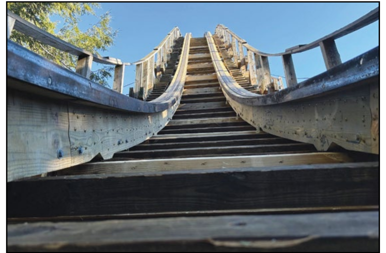
Funtown management report the off-season track work has increased the speed of Excalibur. Major curves received needed attention (above middle). In addition, Excalibur's first drop (above right, below) received precut track from The Gravity Group. COURTESY FUNTOWN SPLASHTOWN U.S.A., THE GRAVITY GROUP
