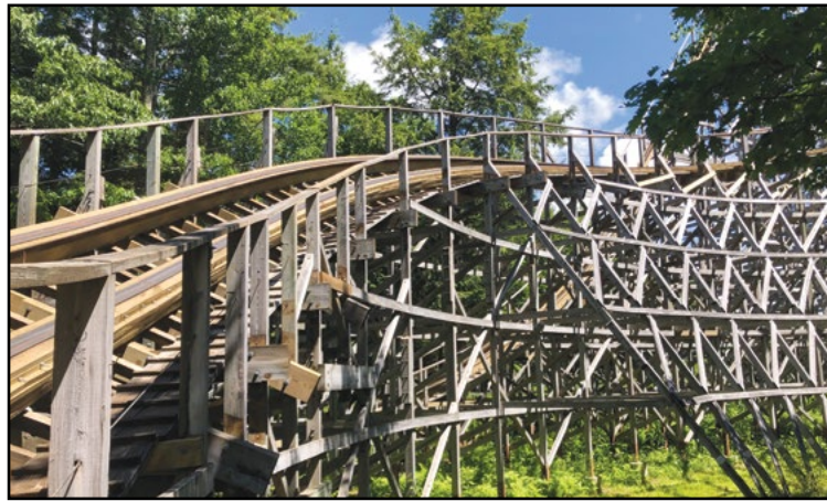
Excalibur's rehab work has it running in top form. The vertically stacked track is seen with a label from The Gravity Group (above right). COURTESY FUNTOWN SPLASHTOWN U.S.A.
