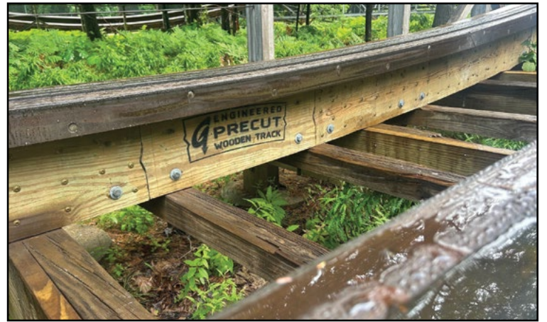
Excalibur's rehab work has it running in top form. The vertically stacked track is seen with a label from The Gravity Group (above right). COURTESY FUNTOWN SPLASHTOWN U.S.A.
