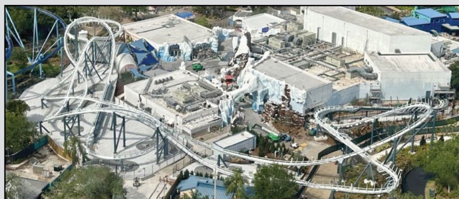
Penguin Trek is a 65-foot-tall, 3,020-foot-long roller coaster which reaches speeds of up to 43 mph. COURTESY SEAWORLD ORLANDO
