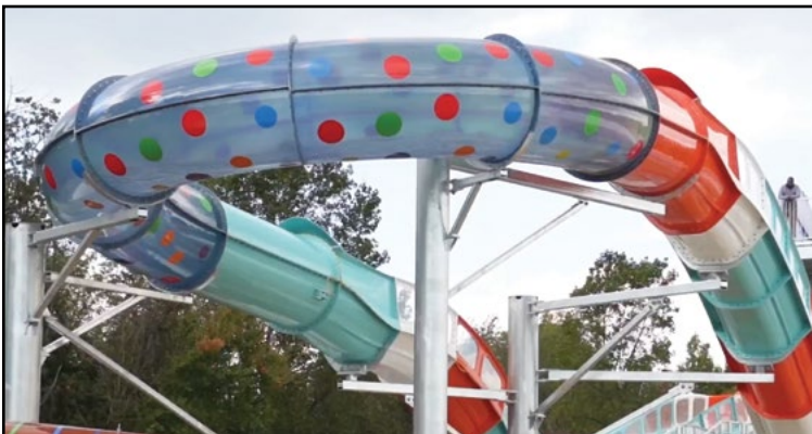
AquaLucent tube sections allow the slide to be illuminated with natural sunlight. COURTESY HURRICANE HARBOR MARYLAND
