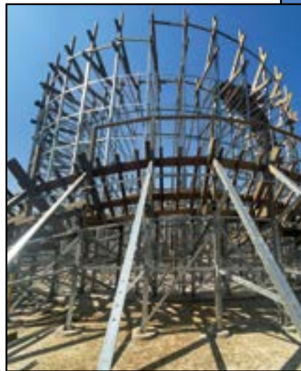
The layout features numerous banked curves, a trademark of GCII designs. Steel structure with wood track is a first for a coaster in China (below). COURTESY GCII
