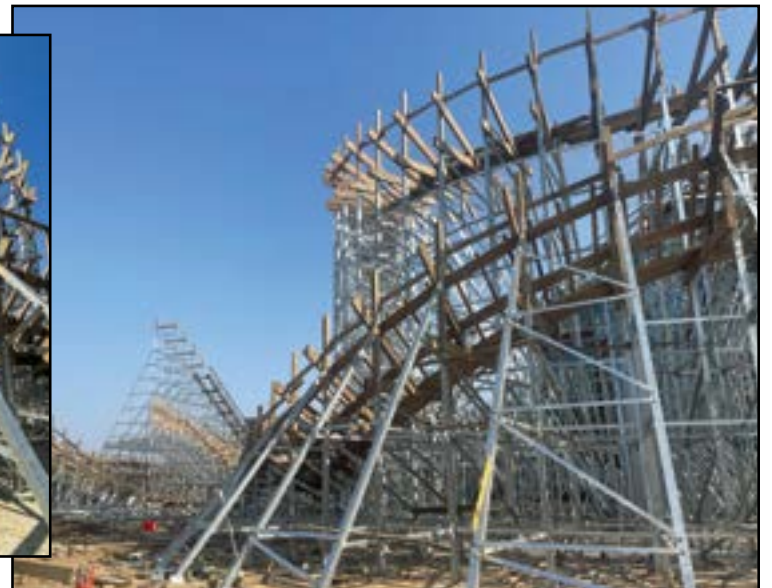
The layout features numerous banked curves, a trademark of GCII designs. Steel structure with wood track is a first for a coaster in China (below). COURTESY GCII
