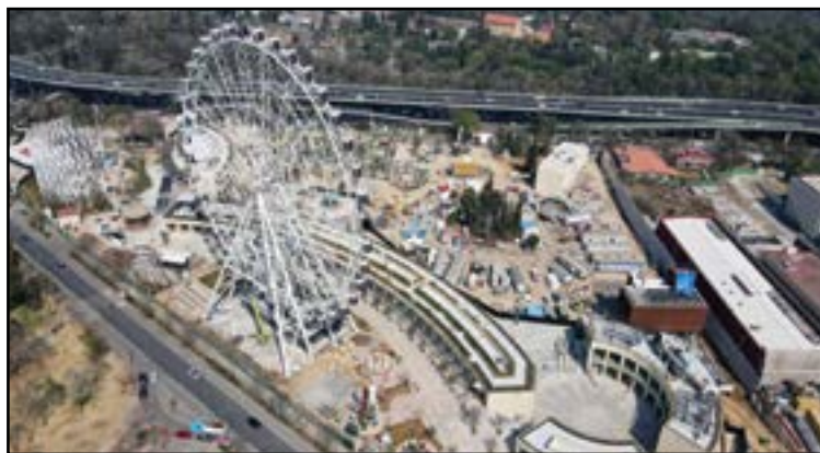
This construction overview (above) shows the curved sculpture of the former wooden coaster, now a monument in steel. The new 85-meter — 279-foot — wheel from Fabbri is a new icon for Mexico City (right). COURTESY AZTLÁN PARQUE URBANO
