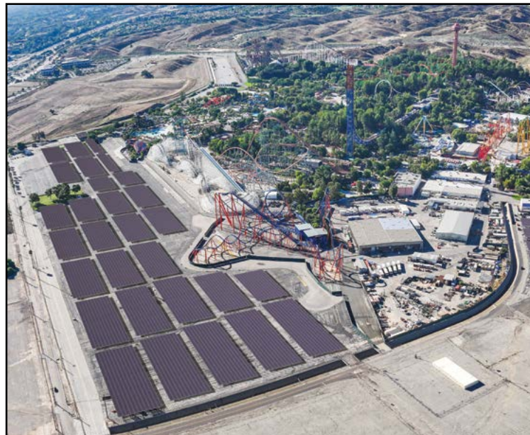
Six Flags Magic Mountain has broken ground on a 637,000-square-foot, 12.37-megawatt solar carport over the main guest parking lot and team member parking lot. With it, the park will be able to offset 100% of its energy usage with solar power. COURTESY SIX FLAGS
