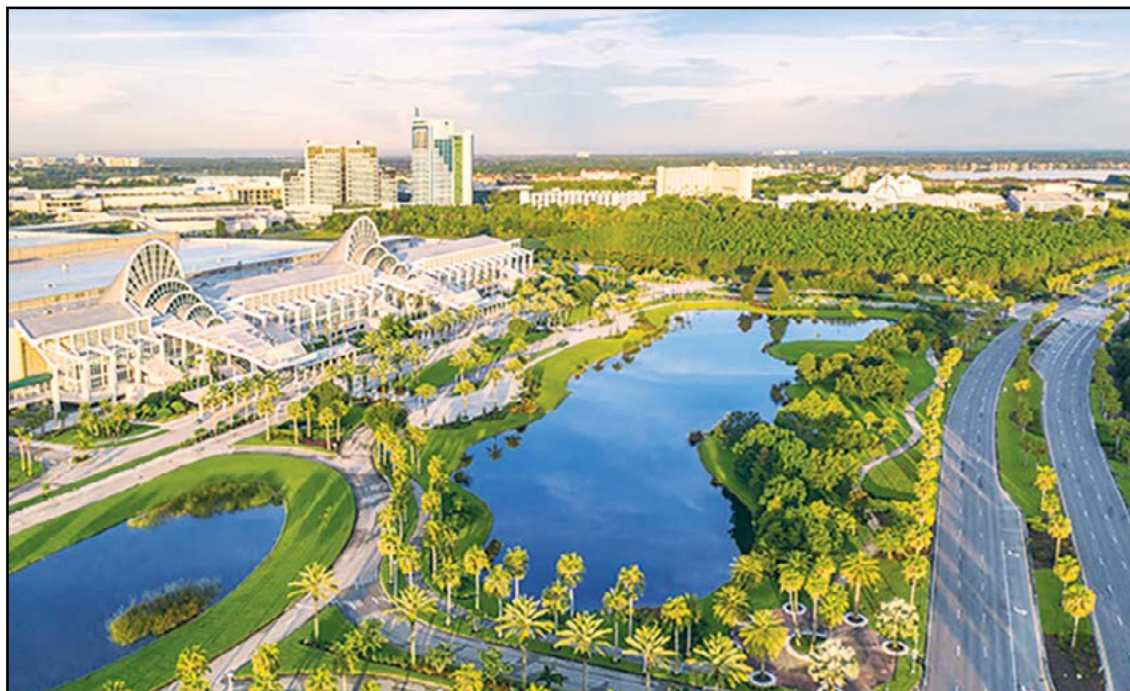
The Orange County Convention Center is a leader in its sustainability efforts and was awarded the Gold Level of Leadership in Energy and Environmental Design certification in 2013. COURTESY OCCC
