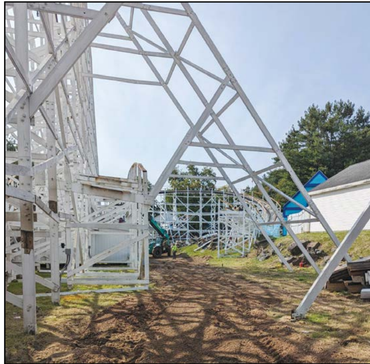
Palace has opted for the restoration of Wildcat to be a completely wood solution provided by The Gravity Group. A total restoration of sections of track are taking the coaster down to the footings. COURTESY PALACE ENTERTAINMENT
