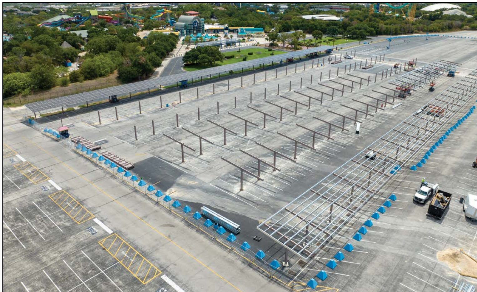
Seaworld San Antonio, Texas, began construction last month on its new solar canopy. The canopy will provide shade for 1,200 cars and will produce 16% of the park's electricity consumption. COURTESY SEAWORLD SAN DIEGO
