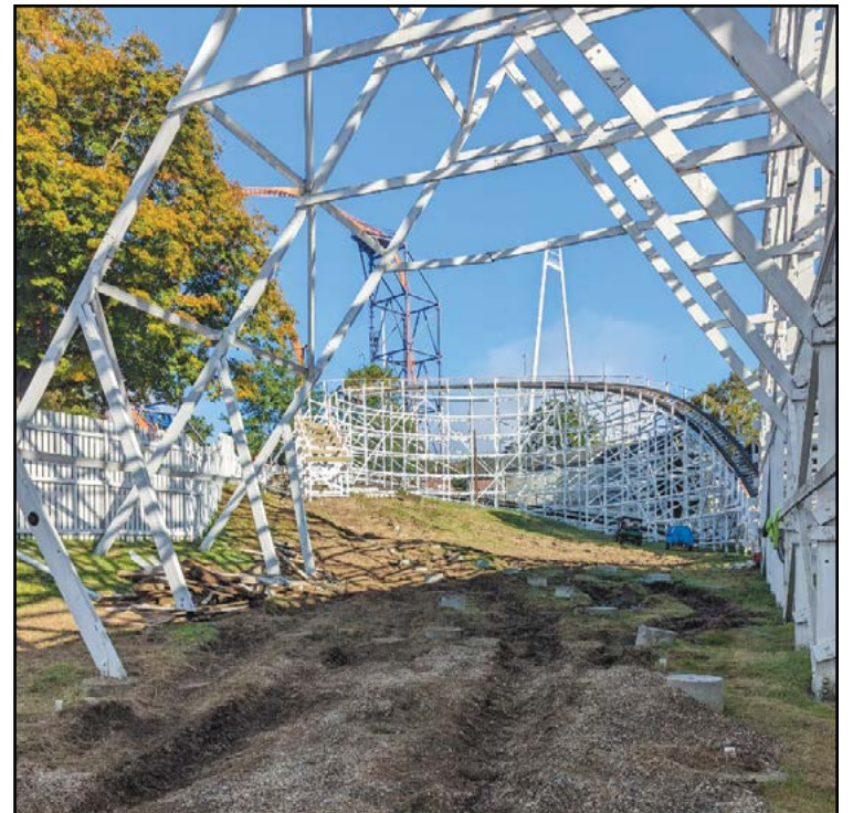
Palace has opted for the restoration of Wildcat to be a completely wood solution provided by The Gravity Group. A total restoration of sections of track are taking the coaster down to the footings. COURTESY PALACE ENTERTAINMENT
