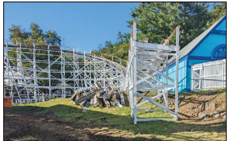
Palace has opted for the restoration of Wildcat to be a completely wood solution provided by The Gravity Group. A total restoration of sections of track are taking the coaster down to the footings. COURTESY PALACE ENTERTAINMENT
