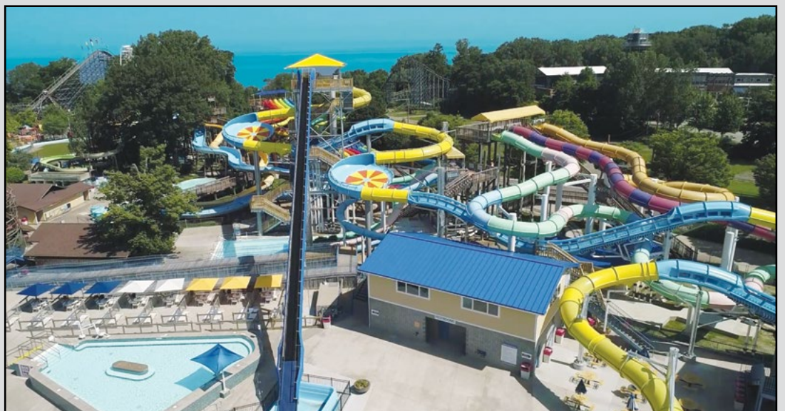
The aerial view shows how Rocket Blast had to be carefully fitted over and under the park's existing slides. COURTESY WALDAMEER & WATER WORLD
