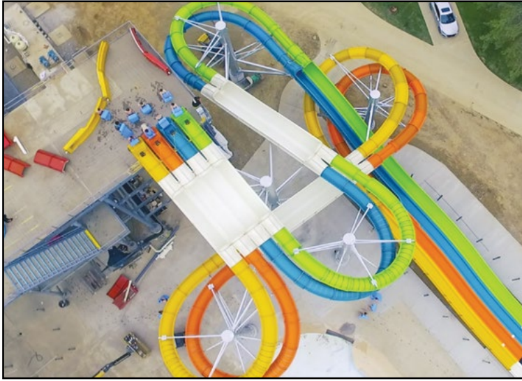
As seen from above, the left pair and right pair of slides diverge onto different paths following the first rally point. COURTESY NASHVILLE SHORES
