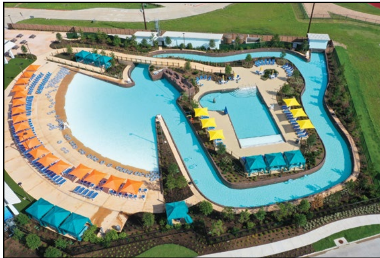
The wave pool, tidal river and activity pool at Meridiana, are for the exclusive use of residents of the master-planned community. COURTESY ADG
