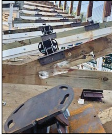
The difference between RMC's Topper Track and their 208 ReTraK is that the Topper Track still maintains a wood element. COURTESY FUN SPOT AMERICA
