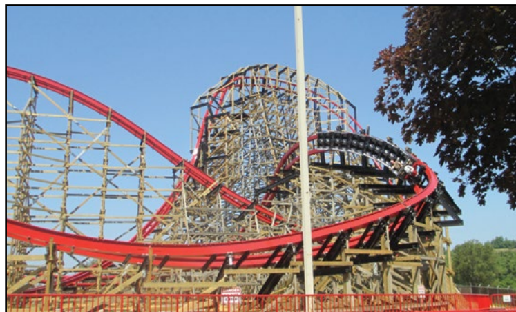
The original footers and a third of the GCII structure were used in the reprofiled model (above). Wildcat's Revenge is the latest coaster at Hersheypark. This is the first time RMC has done any work in Pennsylvania. COURTESY HERSHEY PARK; AT/B. DEREK SHAW
