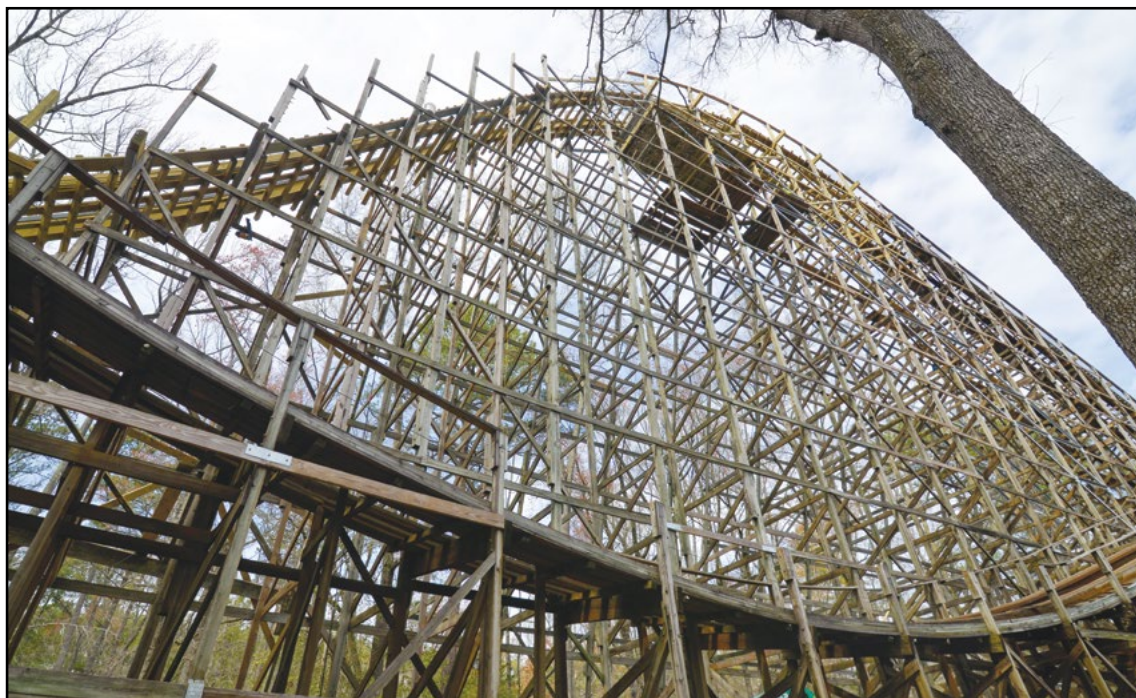
The newly refurbished Grizzly wooden roller coaster has come back with a roar at Kings Dominion, Doswell, Virginia. Aside from the retracking, structural changes also were made, including the lowering of the first drop creating a steeper descent and changes to the fan turn to create a smoother transition. COURTESY KINGS DOMINION
