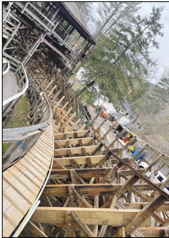
Knoebels' Twister roller coaster saw an entire retrack of its helix, courtesy of Amuse (above left). Amuse worked on California's Great America's Gold Striker to keep it in top form (above right). COURTESY AMUSE
