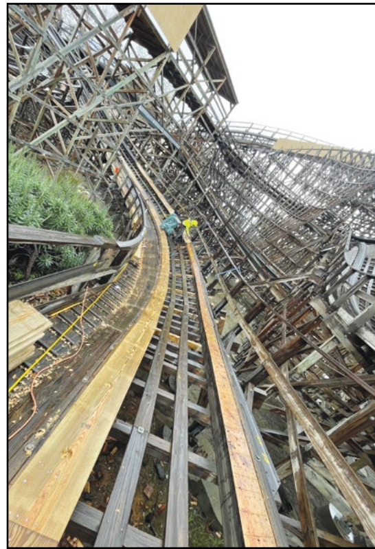
Knoebels' Twister roller coaster saw an entire retrack of its helix, courtesy of Amuse (above left). Amuse worked on California's Great America's Gold Striker to keep it in top form (above right). COURTESY AMUSE
