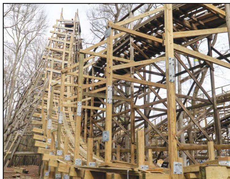
The newly refurbished Grizzly wooden roller coaster has come back with a roar at Kings Dominion, Doswell, Virginia. Aside from the retracking, structural changes also were made, including the lowering of the first drop creating a steeper descent and changes to the fan turn to create a smoother transition. COURTESY KINGS DOMINION
