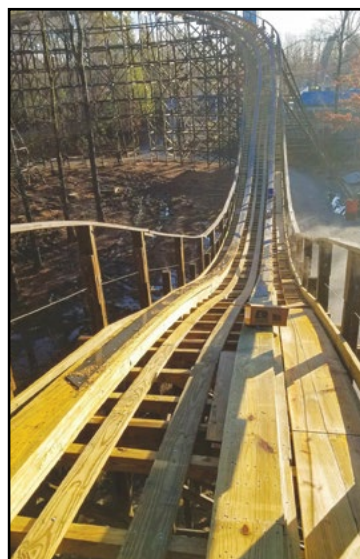
The coaster, which originally opened in 1982, reopened on May 13, 2023. It was designed by Curtis D. Summers and built in-house by Kings Dominion staff. The Grizzly has had over 1,000 feet of track replaced by The Gravity Group, which was contracted to do the refurbishment. COURTESY KINGS DOMINION
