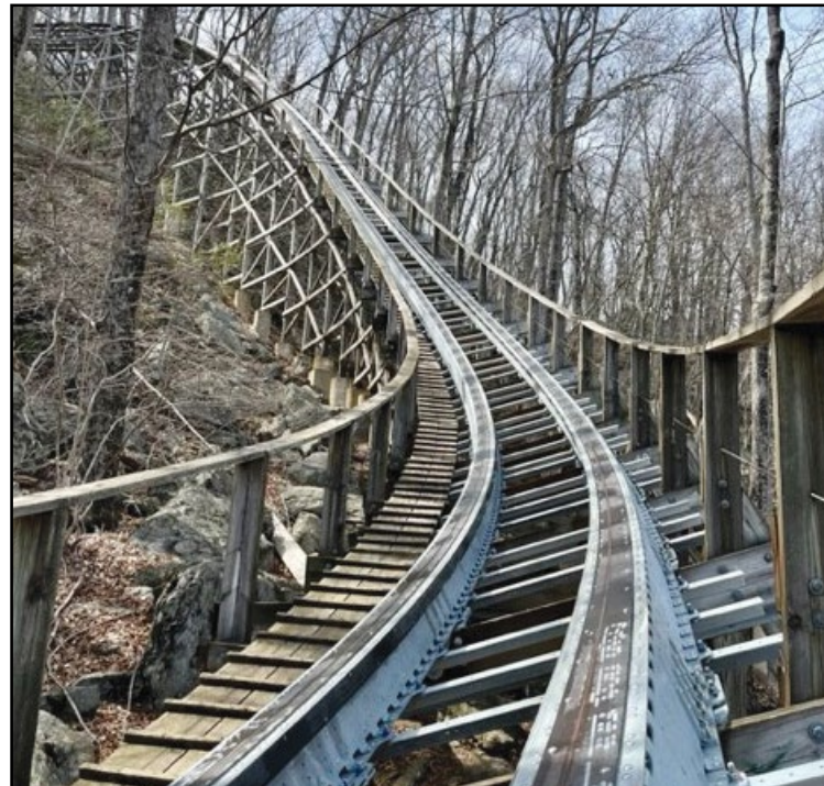
The installation of 580 feet of GCII’s Titan Track (right) will provide a solution to problem areas on Lake Compounce’s popular wooden coaster Boulder Dash (above). COURTESY LAKE COMPOUNCE, GCII
