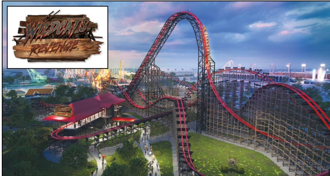
A new lift truss system will increase the ride's height to 140 feet. COURTESY HERSHEY PARK
