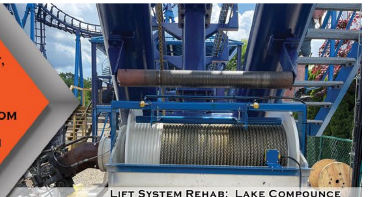
LIFT SYSTEM REHAB: LAKE COMPOUNCE
