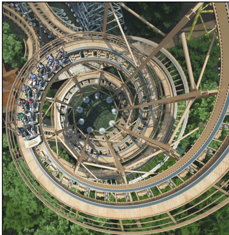
The spiral lift of the original ride is being recreated in the new version — a first for a wooden coaster. The new version will stand 17 feet taller than the original. COURTESY WORLDS OF FUN
