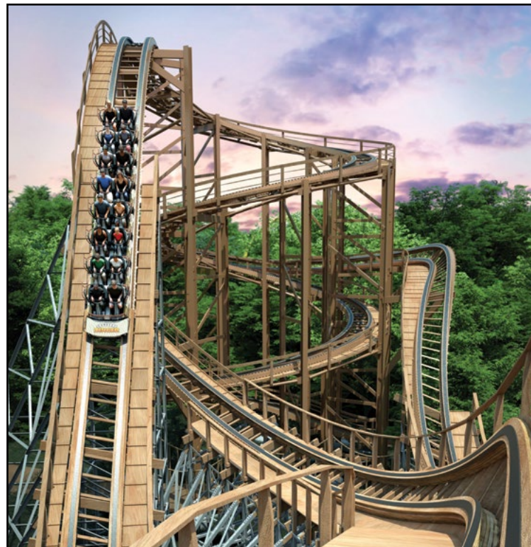
The spiral lift of the original ride is being recreated in the new version — a first for a wooden coaster. The new version will stand 17 feet taller than the original. COURTESY WORLDS OF FUN
