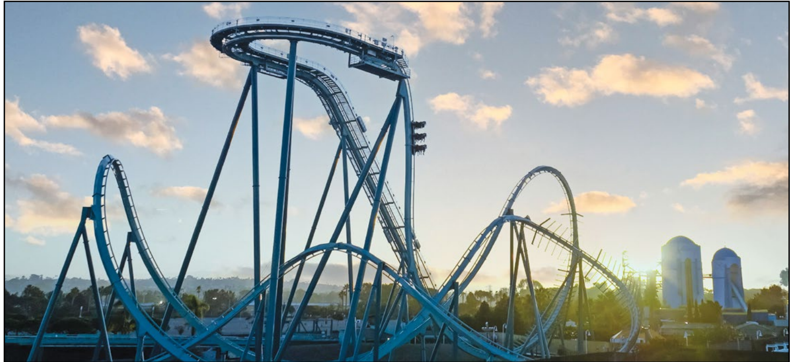
The much-anticipated new Emperor dive coaster at SeaWorld San Diego opened on March 12. Manufactured by Bolliger & Mabillard, the coaster rises 153 feet into the air and offers a 143-foot vertical drop with riders facing downward. Seating configuration for the coaster is three, six-person cars for a total of 18 riders. COURTESY SEAWORLD SAN DIEGO
