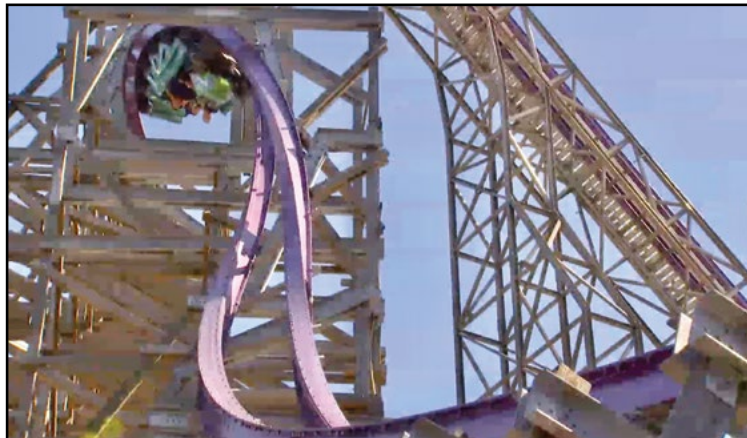
RMC's Alan Schilke-designed coaster, with its durable IBox track hybrid design, utilizes approximately 40% of the structure and track layout of its former incarnation, and original Gwazi footers can be seen while riding Iron Gwazi. AT/DAVID FAKE
