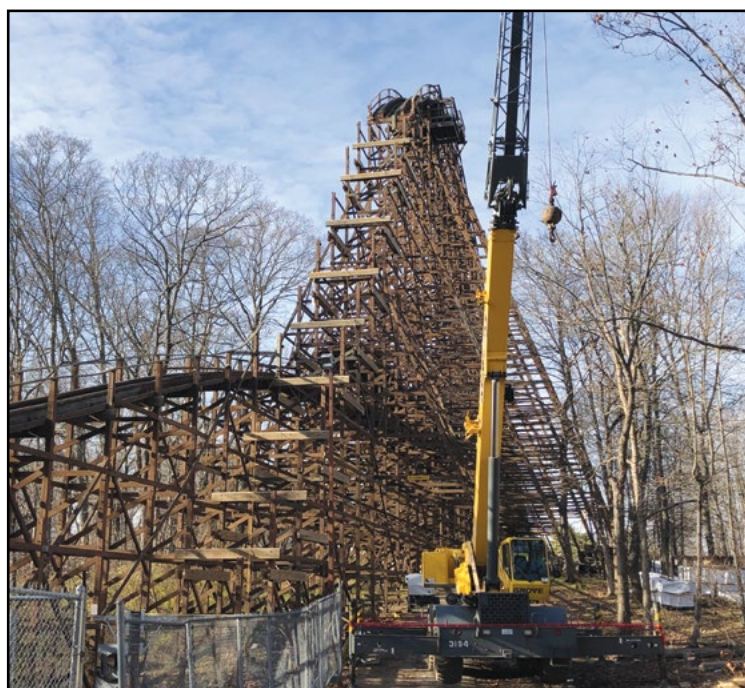
The entire first drop is being retracked at a steeper angle. COURTESY KINGS ISLAND
