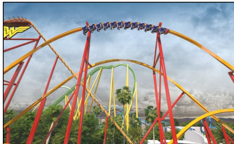
The 20th roller coaster for the park will be a part of the DC Universe section. Wonder Woman Flight of Courage is the second roller coaster from Rocky Mountain Construction at Magic Mountain. The single-rail coaster features three inversions and numerous moments of airtime. COURTESY SIX FLAGS MAGIC MOUNTAIN
