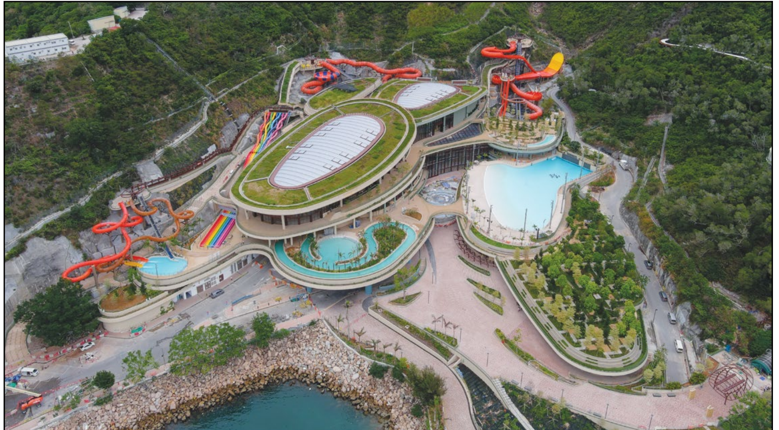
These aerial views show the massive ETF skylight system surrounded by a green roof as well as the multiple levels and careful placement of each attraction. COURTESY OCEAN PARK WATER WORLD
