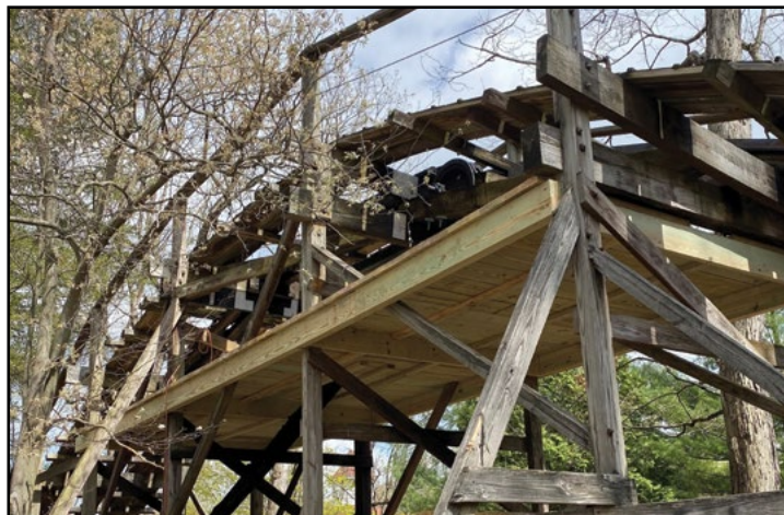
One of the safety benefits to the work on Idlewild's Rollo Coaster is the addition of an inspection platform on the lift hill. COURTESY AMUSE RIDES
