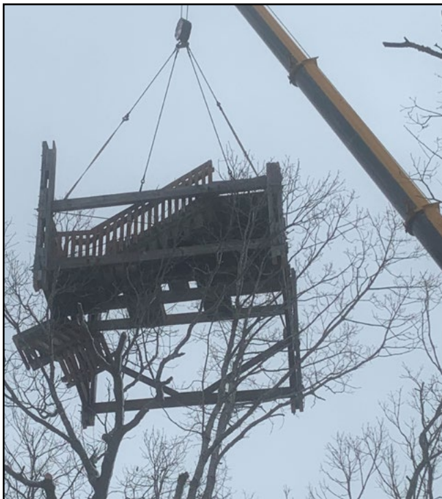
Splish Splash required several days to work on repairing slide structures, removal of a slide tower and the addition of new staircases. COURTESY AMUSE RIDES
