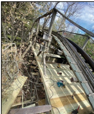
One of the safety benefits to the work on Idlewild's Rollo Coaster is the addition of an inspection platform on the lift hill. COURTESY AMUSE RIDES
