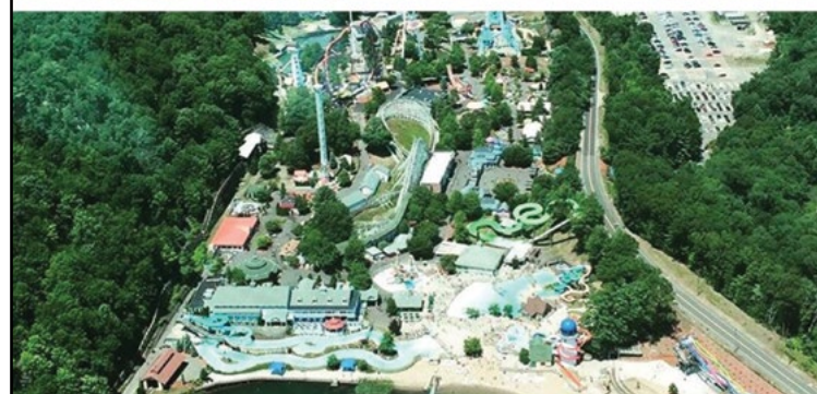
Above is an overview of Lake Compounce, showing the changes over the years. In the older photo (top), the parking lot was directly adjacent to the Wildcat. COURTESY LAKE COMPOUNCE
