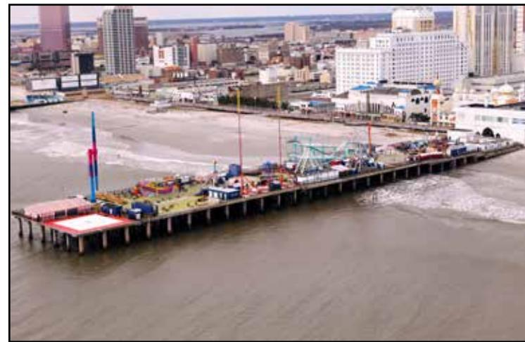
to support a proposed casino hotel, is a concrete deck built upon 10-foot-diameter concrete pilings reinforced with baseball bat-thick rebar and driven 100 feet into the seabed.
