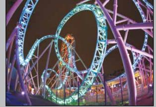
KCL's lighting package for HangTime offers a rainbow of programmable color combinations, as well as a variety of motion effects. **COURTESY KCL ENGINEERING**
