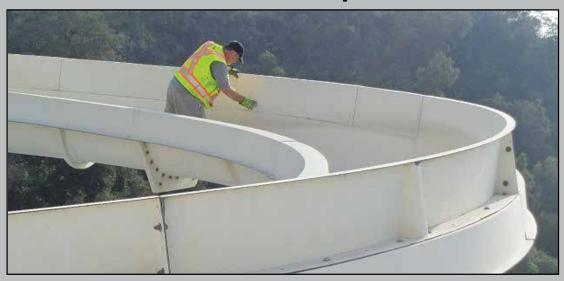
Mike Nicol, LJM & Associates, Inc., is seen here performing the QSI (Qualified Safety Inspector) Annual Inspection on a waterslide at the Raging Waters water park in the Los Angeles area. During the QSI, the inspector will look for wear/spider cracks in the fiberglass and gel-coating; check all the stairways, structural items, towers, columns and footings and check all the operational systems of the slide. COURTESY LEWIS MERZ/LJM & ASSOCIATES, INC.
