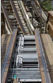
Lagoon's carpentry and maintenance team that worked on Roller Coaster posed for a photo. Magnetic brakes (right) now bring the trains to a smooth stop upon returning to the station. COURTESY LAGOON; AT/TIM BALDWIN
